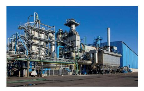
Complete flue gas cleaning system downstream from a special waste incineration plant with waste heat boiler and steam turbine
