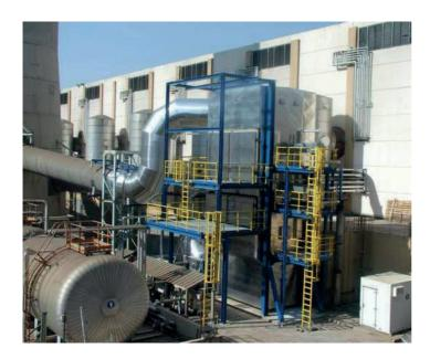
DeNOx- system for the reduction of the nitrogen oxide (NOx) from the exhaust gases from heavy oil diesels
